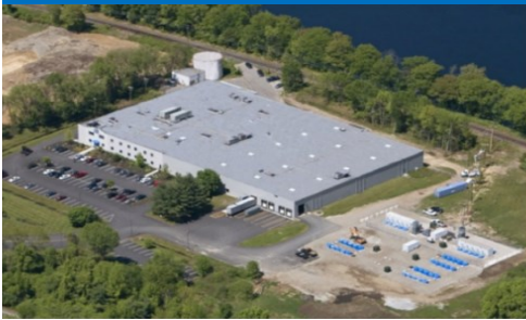
Tyngsboro, MA, 0.5 MW Operating since 2008
